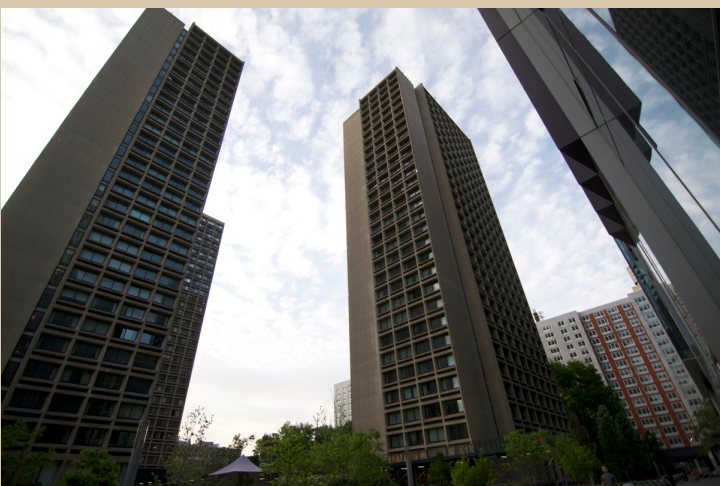
Above: University Village Silver towers in the front and Washington Square Village behind
