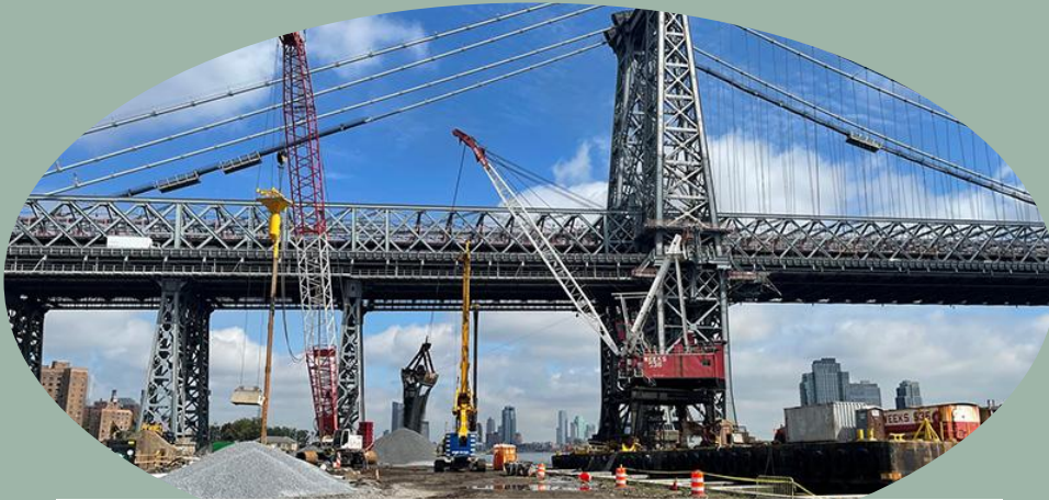
Construction of the ESCR project under the Williamsburg Bridge in September 2022
